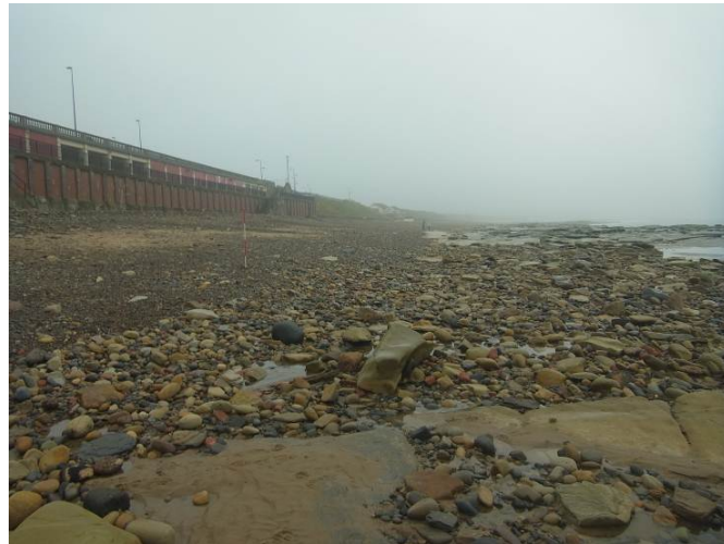
Plate 10 – Survey photograph 1aNTDC04A_20140402_N2
