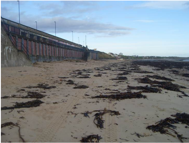
Plate 7 – Survey photograph 1aNTDC04A_20120928_N2
