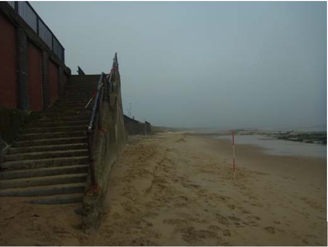
Plate 12 – Survey photograph 1aNTDC04A_20150319_N1
