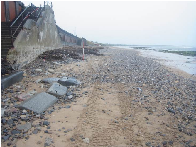
Plate 11 – Survey photograph 1aNTDC04A_20141006_N2
