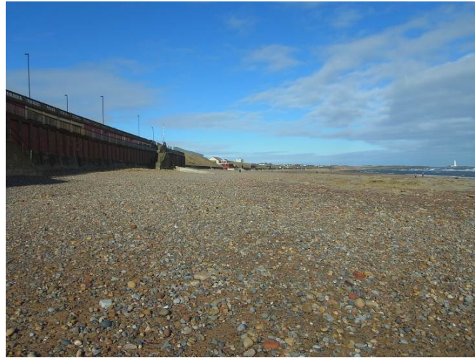
Plate 8 – Survey photograph 1aNTDC04a_20130312_N2
