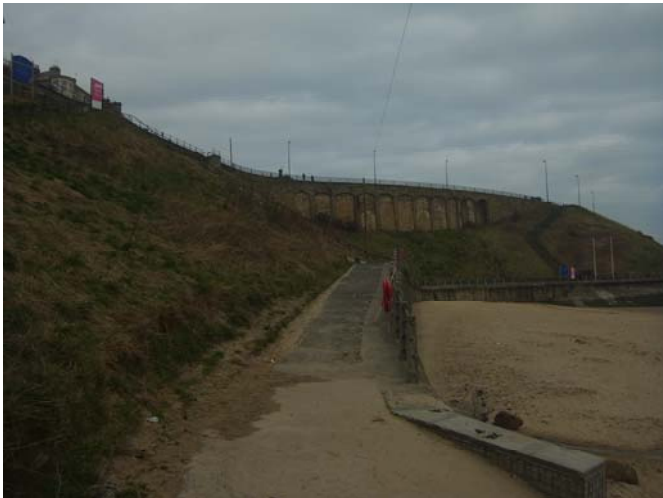
Plate 17 – Survey photograph 1aNTDC08_20150320_N1.JPG
