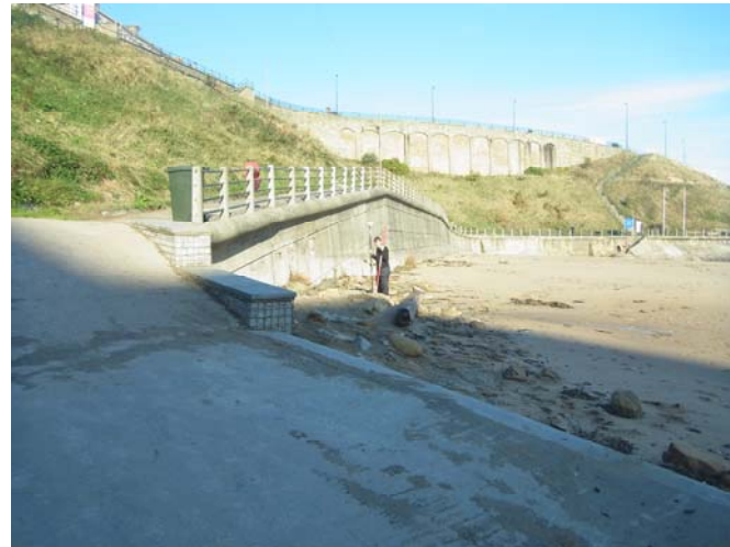
Plate 18 – Survey photograph 1aNTDC08_20141007_N2.JPG.
